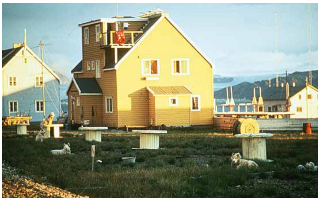
Norwegian Polar Institute's first research station in Ny-Ålesund 15 . In 1989 the former officers mess were enlarged with a third floor and an instrument platform, now gone.
