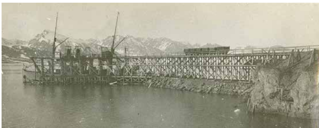
The coal quay in 1925. Today's quay is here 53 . On the quay we can see coal wagons. A ship is being loaded through coal shuts.
